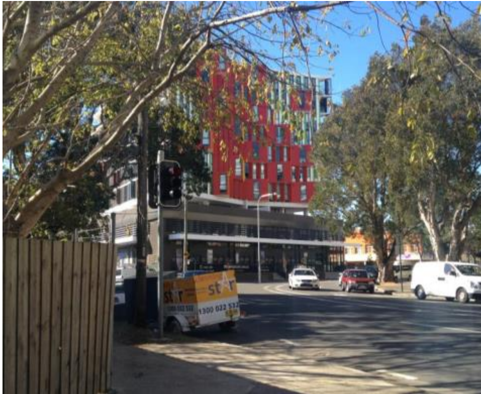
Figure 8: Viking development O'Dea Avenue frontage with subject site on left hand side (timber fence)
